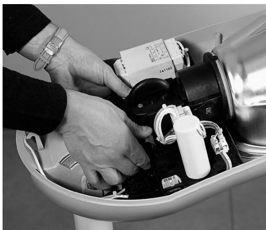
Fig.3 - Lamp replacing
